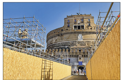
Sites in Rome are under construction for the Jubilee.
