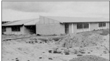
Construction near completion of St Peter's College, July 1974.
