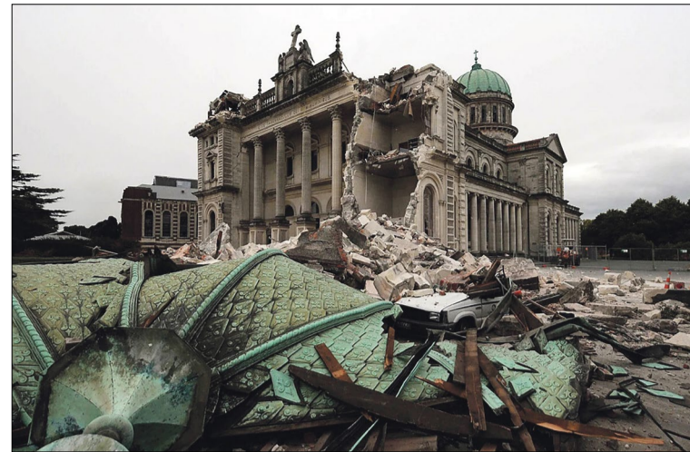
The former Cathedral of the Blessed Sacrament was severely damaged in the 2011 earthquake and was later demolished. Photo: David Wetthey/EPA
