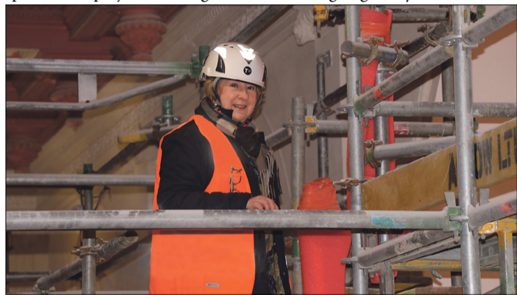
Jane Kelly oversees the restoration work underway. Photo: Supplied
